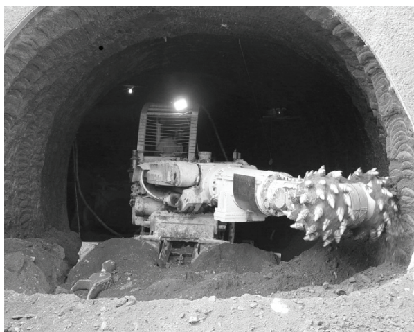
Fig.4 A road header during work procedure
